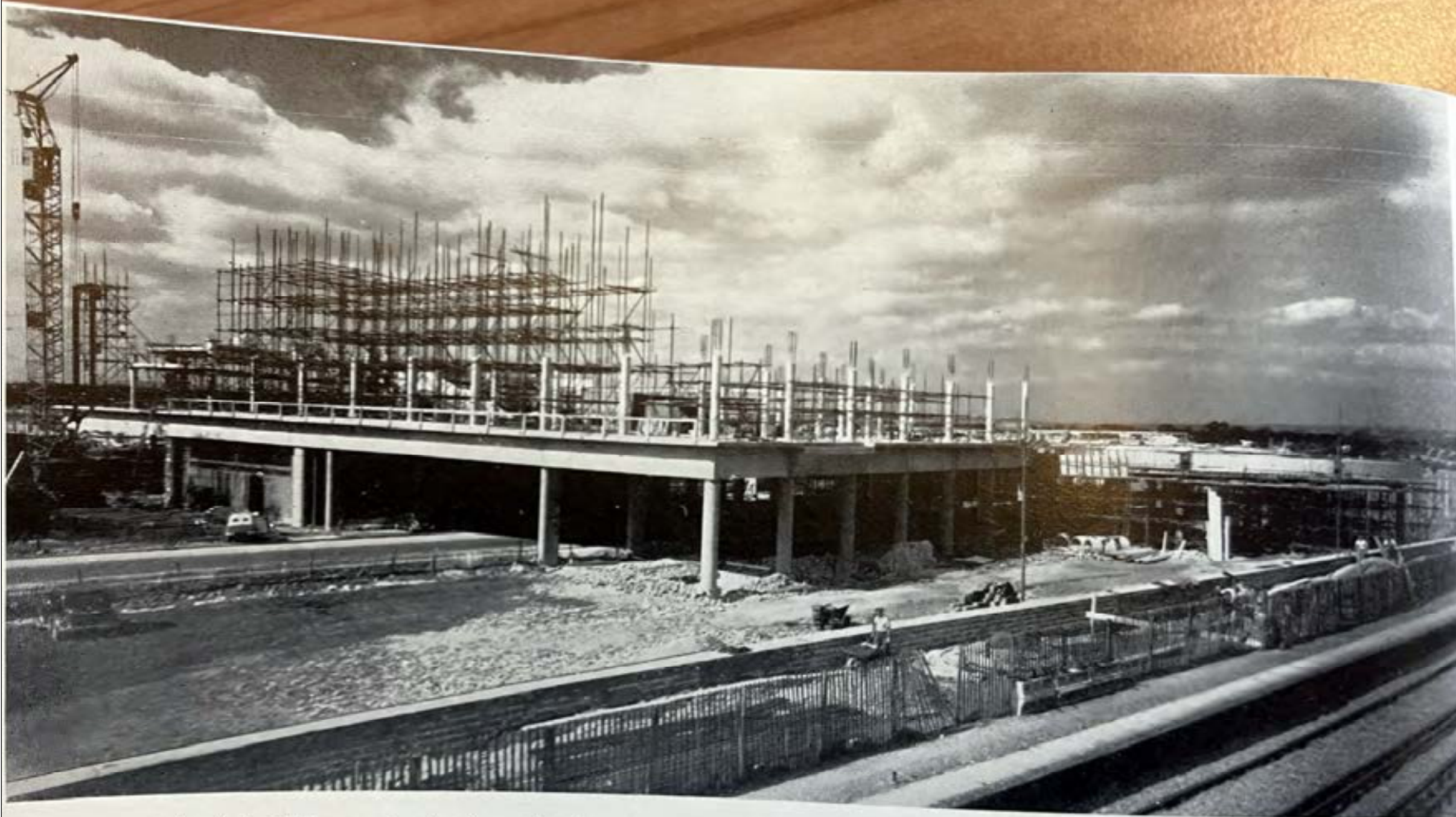
Main terminal building – start of work above concourse level, September 1957
