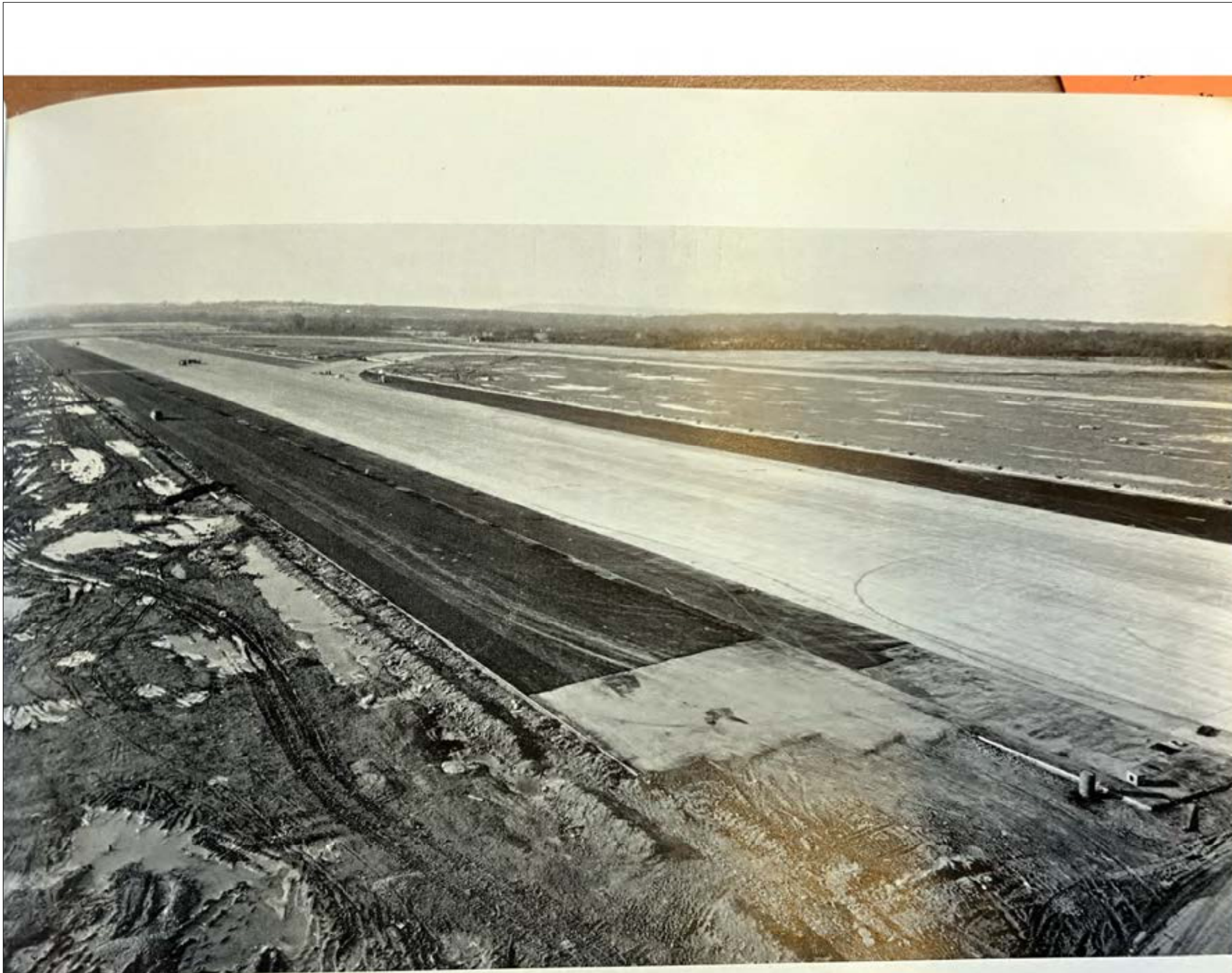
Main runway with shoulder construction proceeding
